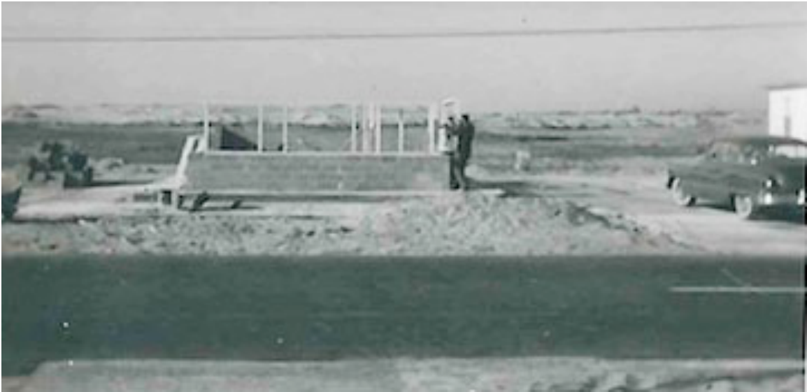
The Dairy Mart under construction
