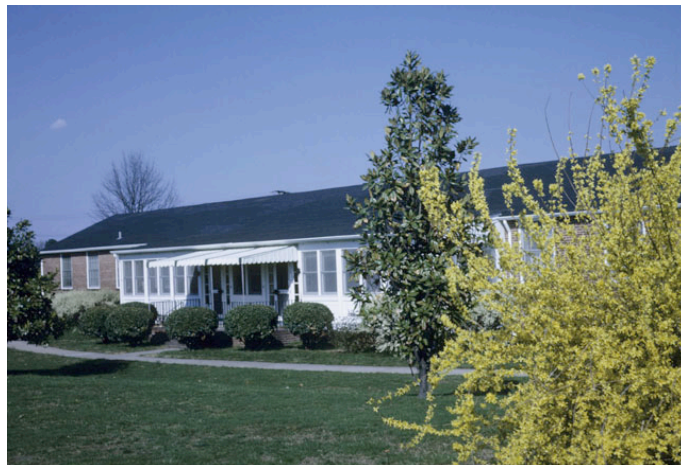
Residence for hospital director (left end) and for director of professional services (right end) (Photo by Jim Scott)
