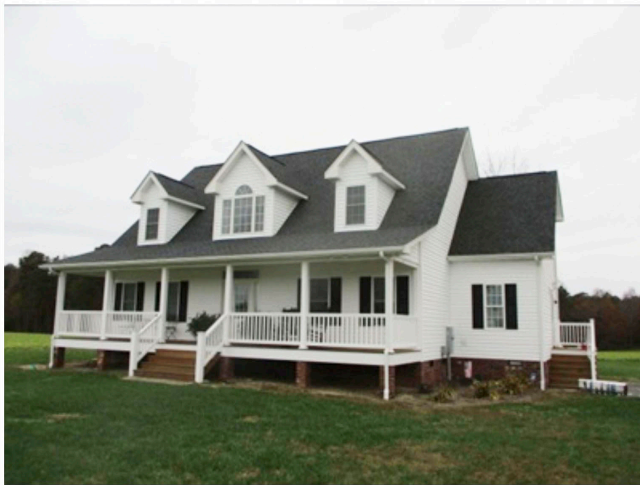
Main Structure Photo
